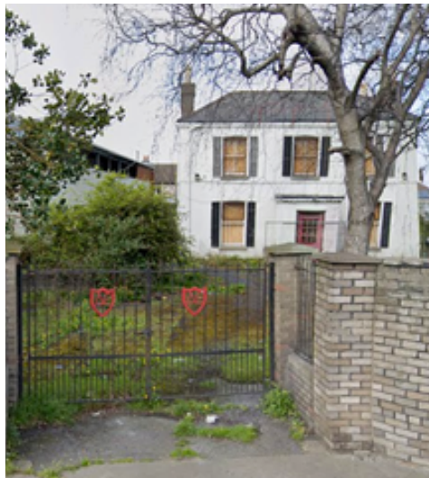
Franshaw House will be renovated for the new library, with an adjacent new building added.
